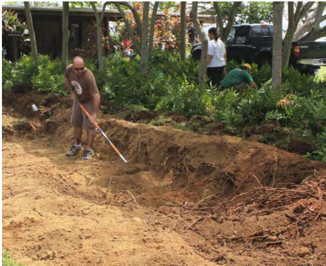
Left: Excavate the rain garden to the proper depth with hand tools and volunteers.
