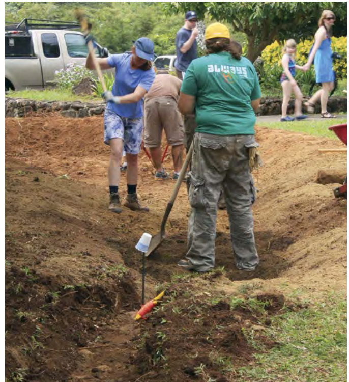
Right: Shape the sides of your rain gardens with hand tools to a minimum 3H:1V slope.
